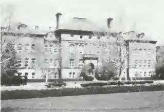
Facade rhythms, Engineering Hall
